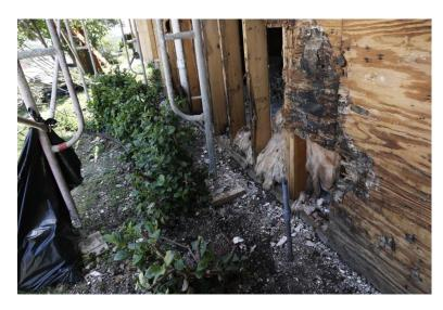
This photo above is particularly interesting. You see that sprinkler head in the foreground? That's the only pipe or penetration I could find anywhere near this massive wall rot area. There was no rot above 4' so the leak wasn't coming from above. Remember that this building is only 10 years old.
